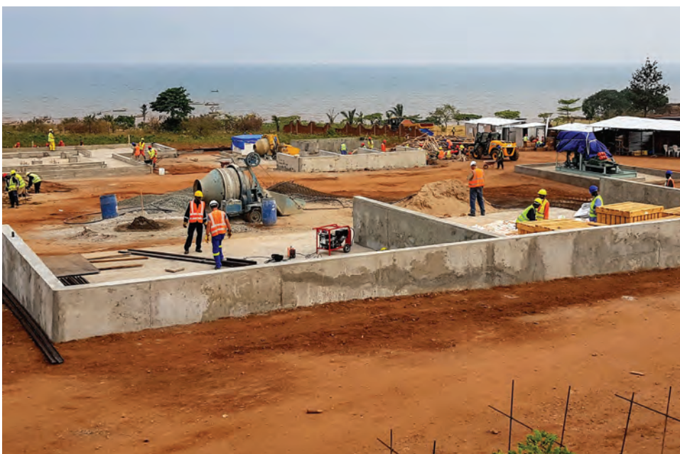
Construction works at Kabezi plant site. September 2017
