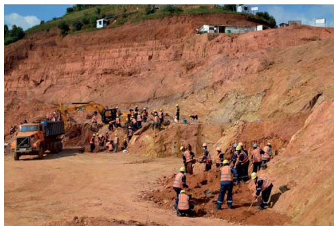
Gasagwe mine site July 2018 (view to north)
