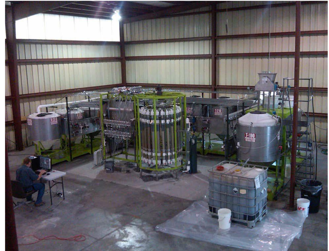
Pilot Plant System for Hydrometallurgical Application
