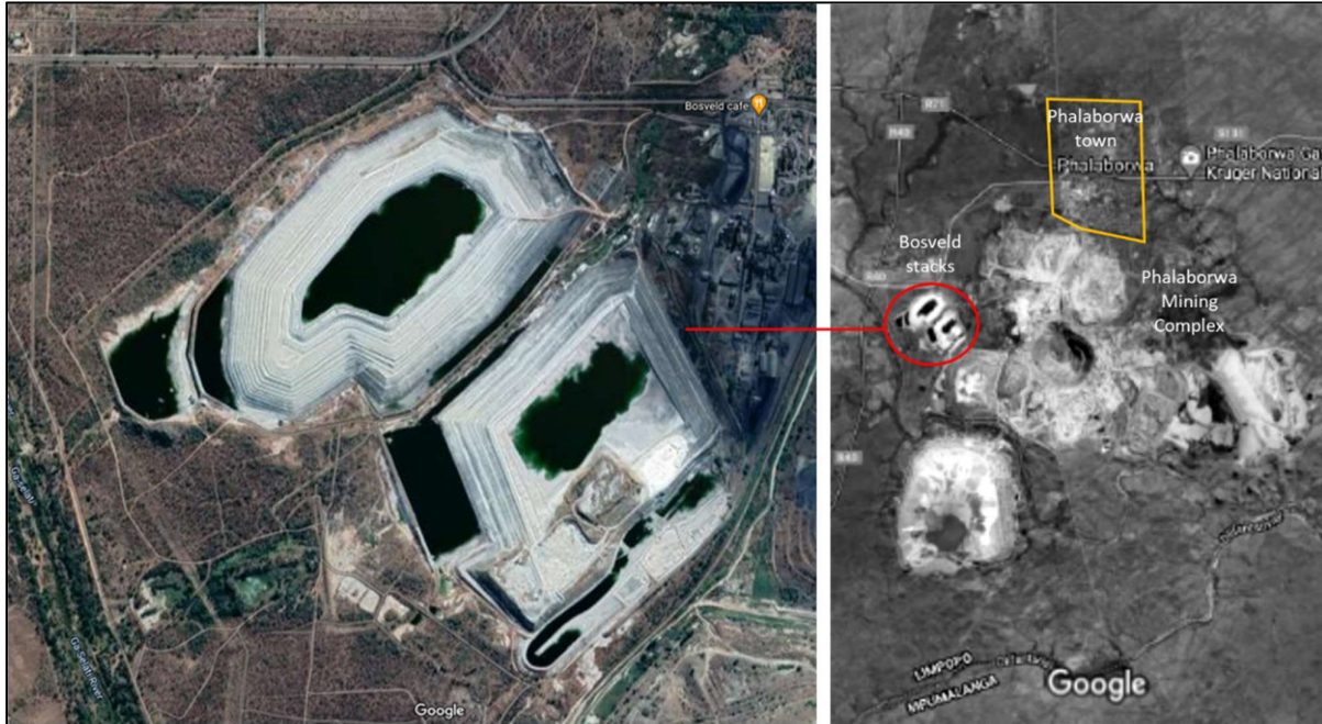
Figure 1.2 Google images of the Bosveld stacks (right –the position of the stacks in relation to the Phalaborwa Mining Complex and town; left – close-up of the stacks annotated as A and B)
