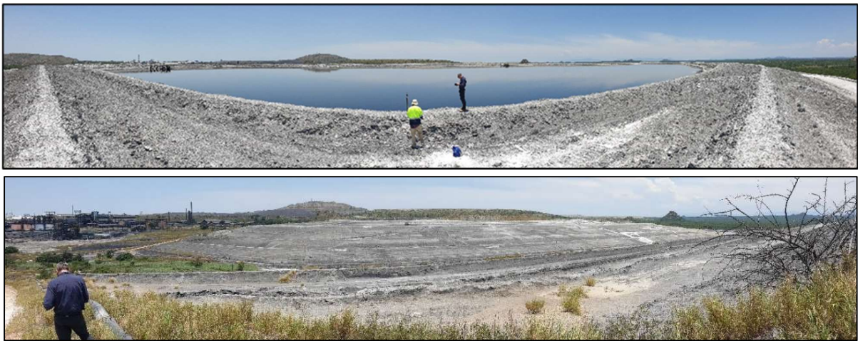
Figure 1.3 View of Stack A (upper) showing existing surface water pond, and Stack B (lower) from Stack A with Phalaborwa Mining Complex in the background
