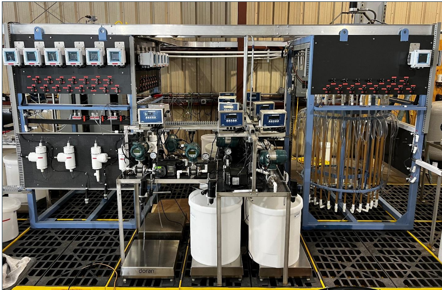
Rainbow's CIX/CIC Units have finished construction and are now being commissioned
